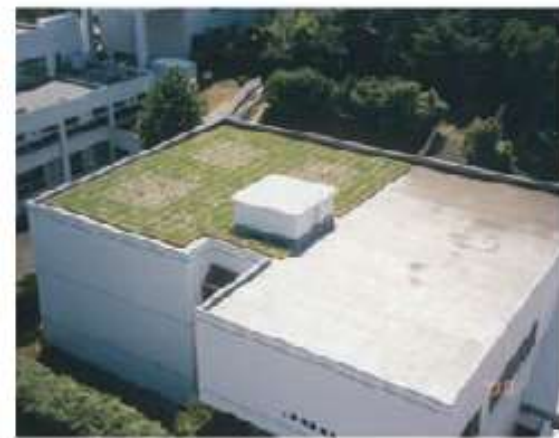
4.47 Experimental green roof on a building (left) at Yokohama National University, Yokohama, Japan. The left side of the roof has pallets of clover, the right side is a conventional exposed roof surface. Infrared thermography (right) shows the effect of the green roof on surface temperatures. ECOTECH LABORATORY
